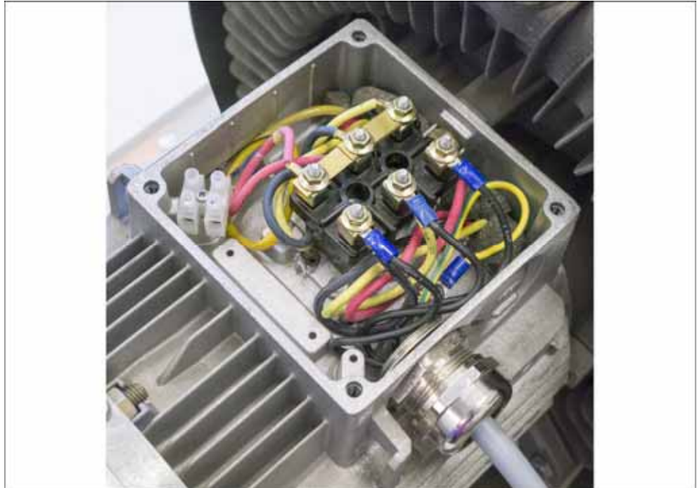
Wiring at the motor connection box
